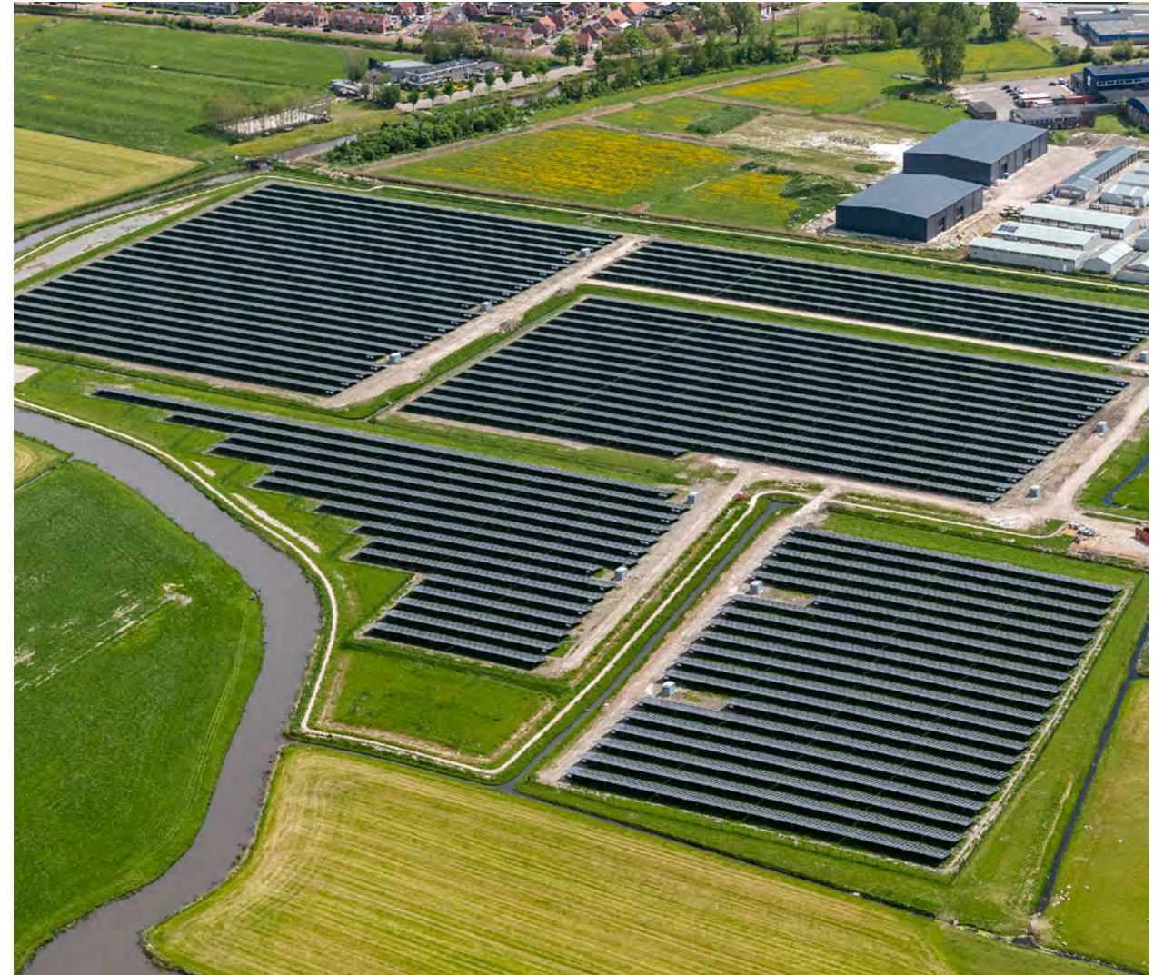
Dokkum solar park (13.9 MW, Netherlands)
