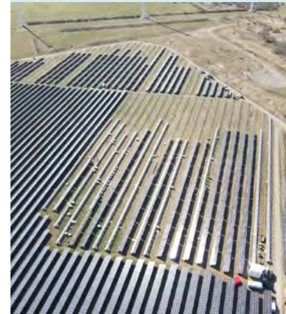
During the conversion
